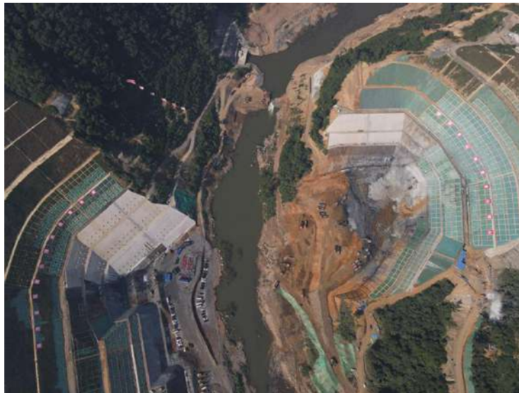
Fig. 1 Slope reinforcement measures for Maiwan Water Conservancy Engineering
