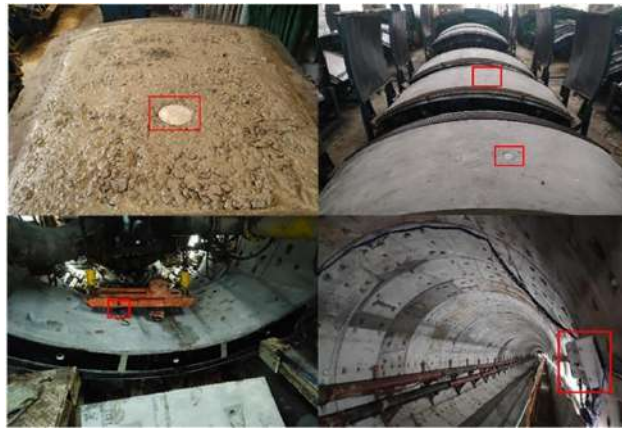
Fig. 1. Preinstallation of pressure cells and field implementation
