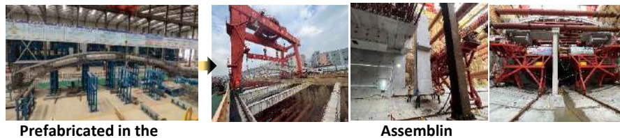
Fig. 1 Photos of the construction process for prefabricated underground station- Longxing station.
